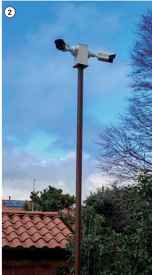
Palo Monaco60 H 4000 mm corten - torretta completa cod. TW5060AB a p. 82
